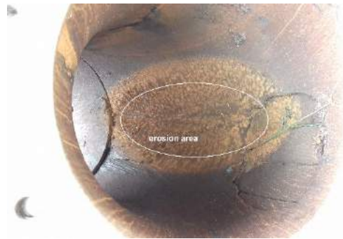
Figure 1. Erosion failure of pulverizer pipe.
